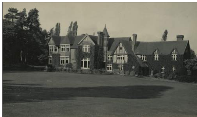
Ivy House, c.1950.
